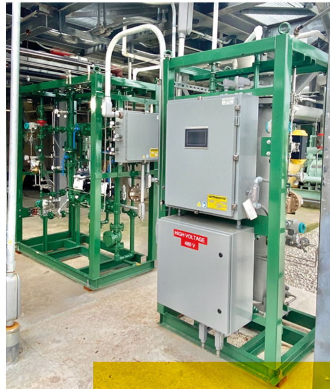
Generator Gas Monitoring and Control Skid (GMCP)
